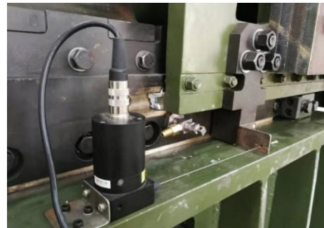
Fig. 5. Displacement sensor installation.
