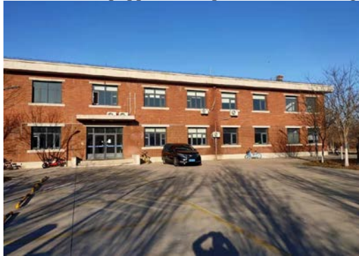
Fig. 1. Realistic scene before renovation.
